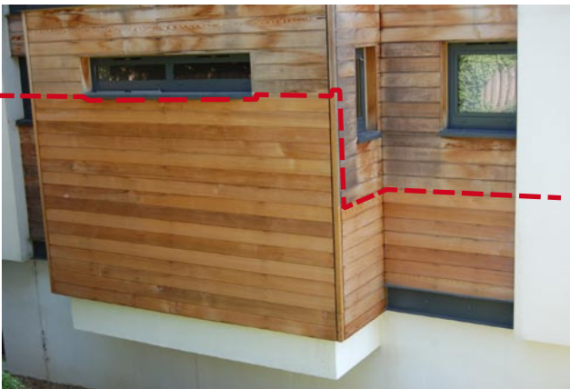
Figure 12 Discoloured western red cedar cladding following cleaning and re-treatment
