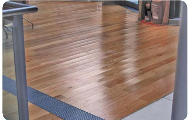
**Figure 1:** Cupping in a timber floor caused by a differential in moisture content between upper and lower faces
