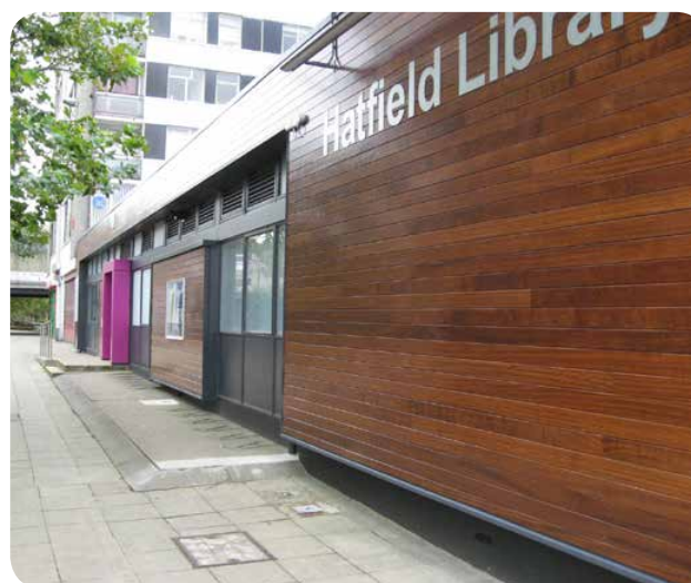
Figure 1: Iroko cladding on Hatfield Library in Hertfordshire Photo: Bryden Wood Associates
