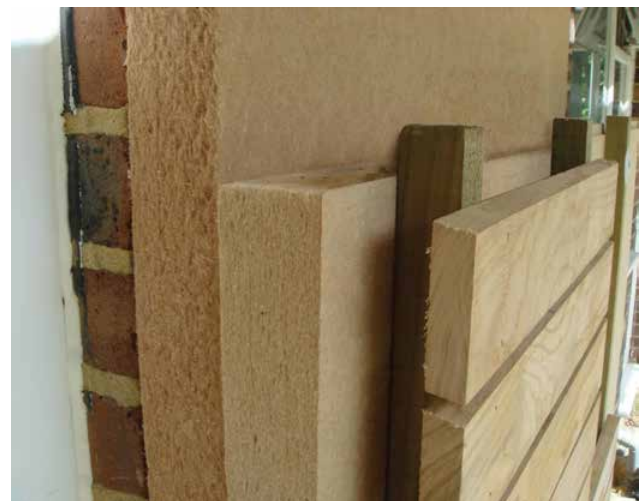
Figure 4: Coppiced sweet chestnut cladding on the Greenhouse in Ripe, East Sussex
