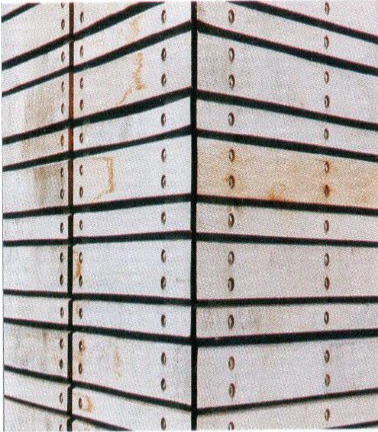
Shadow Gap Mitred Corner details
