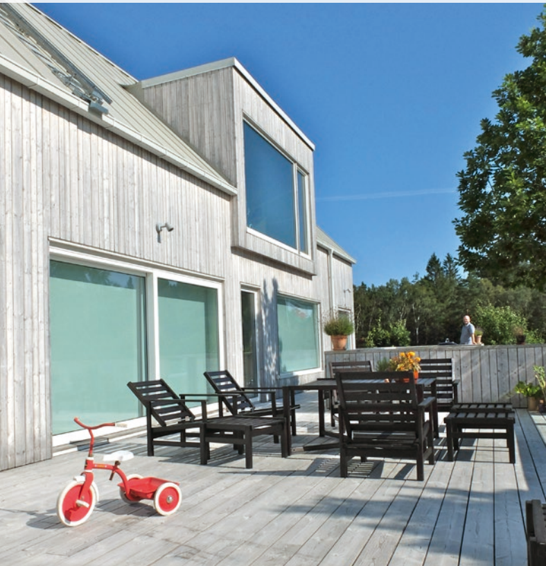
SIOO impregnated spruce. Karlsson Wachenfeldt Architects.
